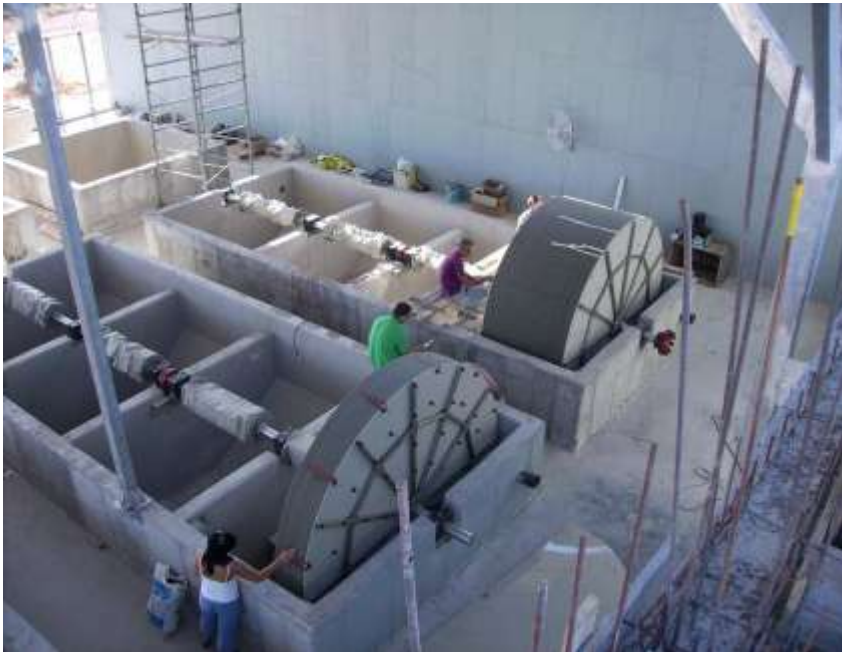
3 m diameter RBC system in Middle East
